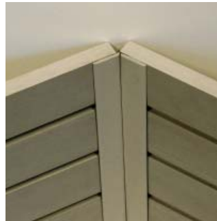
Flat Flat trim can be used to create corners.
