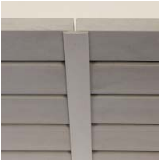
Flat Butt joints
