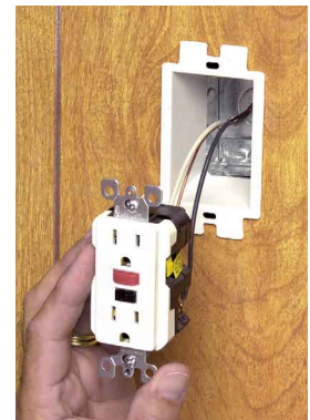
(Option) Turn receptacle on side with wires attached and pass through box extender.
