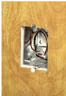
Electrical box is behind the new finished wall surface.
