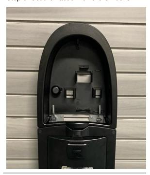
Step 4: Slide the unlocked U-Hook as far over as possible before locking this in place.
